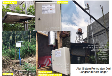
Gambar 3. ( LandSlide Early Warning System (LEWS) )
